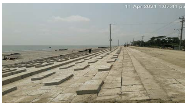
Figure 3-29: Slope Protection work from KM 30+800 to Km 31+450 in Polder-48
