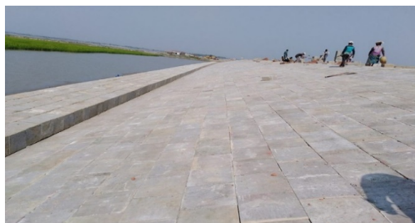
Figure 3-10: Completed Slope Protection Works in Polder-32
