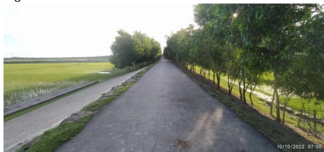
Figure 3-15: Completed Embankment of Polder-32
