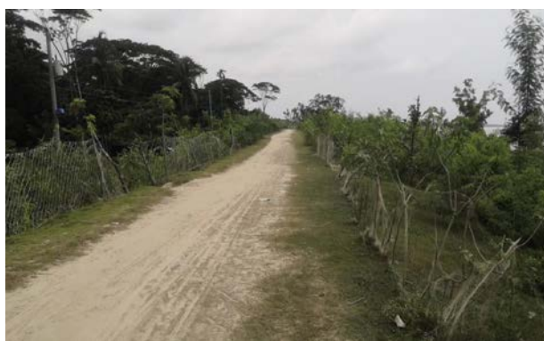
Figure 3-25: Turfing work for k13+100-k15+000 in Polder-40/2
