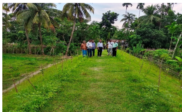
Figure 3-26: Embankment turfing and afforestation work at km 1+170 in Polder-39/2C
