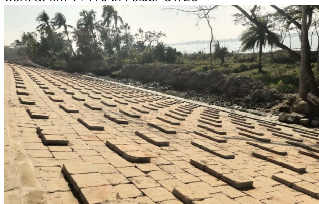
Figure 3-28: Slope Protection work For KM 48+672-48+764 in Polder-39/2C
