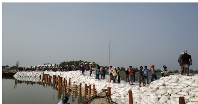
Figure 3-11: Nalian Closure Dam of Polder-32
