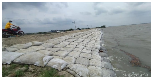
Figure 3-14: Emergency Works of Polder-32
